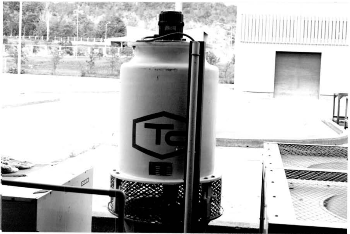
Fig.3.2 Cooling Tower in Model Cooling Tower Systems
