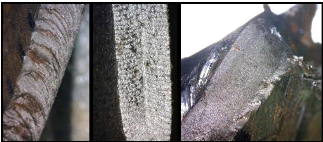
C. Crack surface in propagation, at critical growth and at the beginning (weld-toe).
