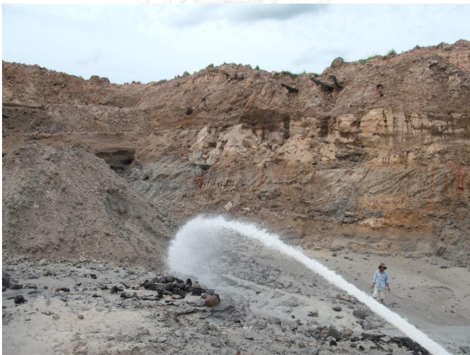
Figure A-3 Water jet stream to leach the sand layer
