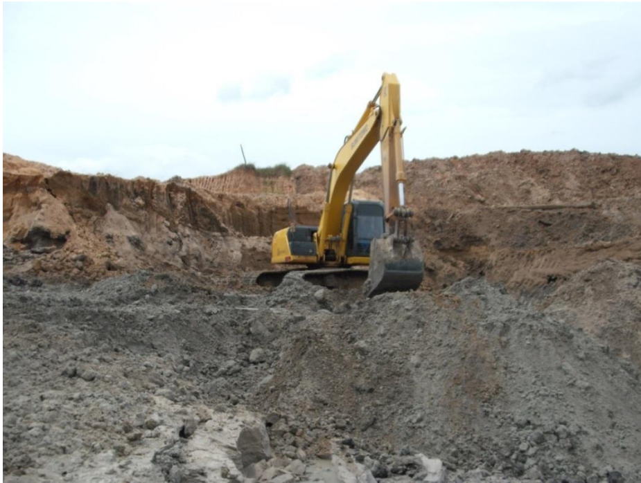
Figure A-2 Backhoe while digging the sand
