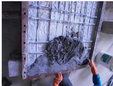
Figure 3.15 Installing the repairing material.
