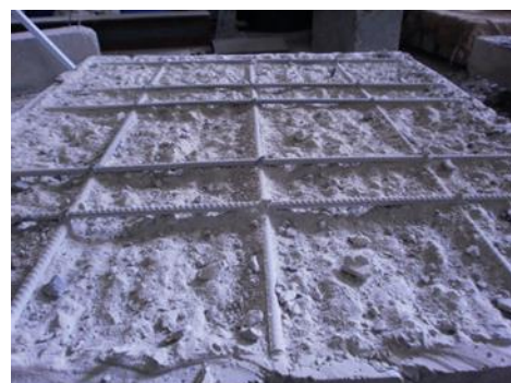
a) Cutting lines on surface of slab b) The surface after removing weakened layer
