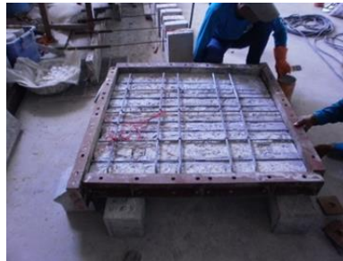
Figure 3.14 Installing steel frame around the slab to cast repairing material.
