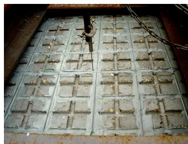
Figure 2.14 NSM rods strengthening in research of Gilles Foret et al [33].
