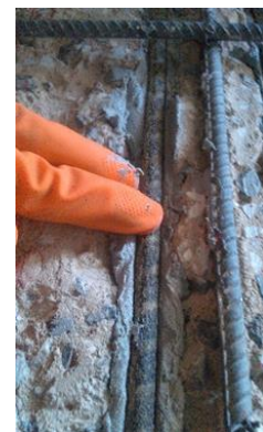
b) Installing CFRP rod into the groove filled with epoxy
