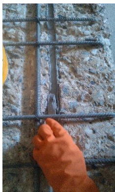
a) Installing epoxy into the groove
