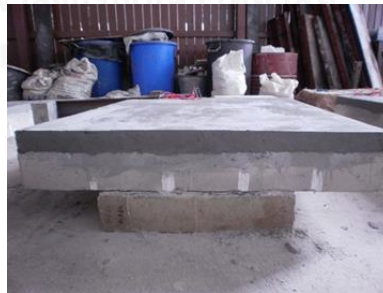
Figure 3.16 The slab after repairing.
