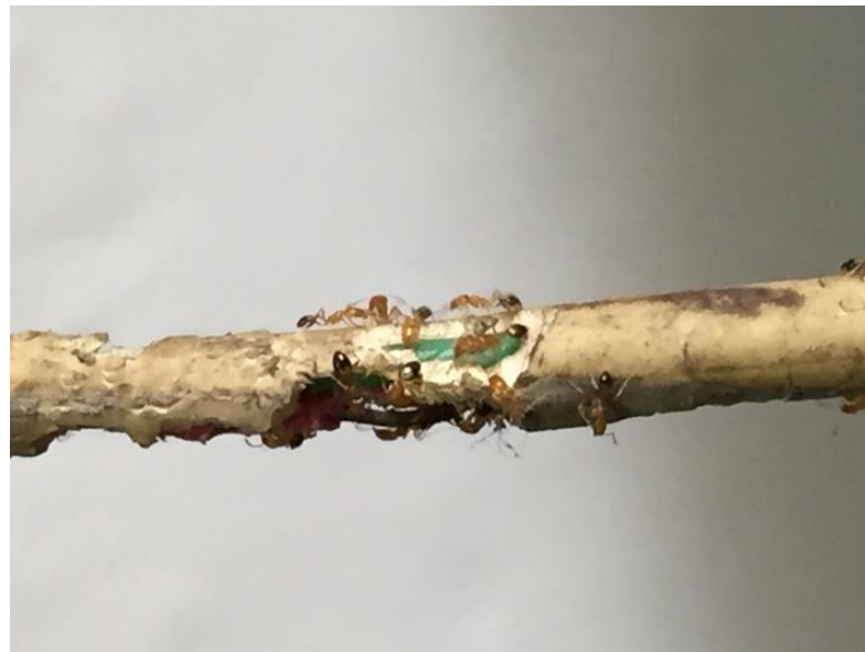
Figure 6 Singapore ants are gnawing electric wire insulation at Biology I Building, Faculty of Science, Chulalongkorn University.
