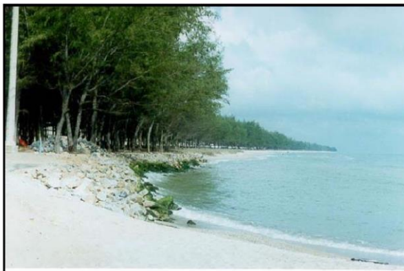
Figure 5 Riprap Seawalls in Chalatat beach, Songkhla
