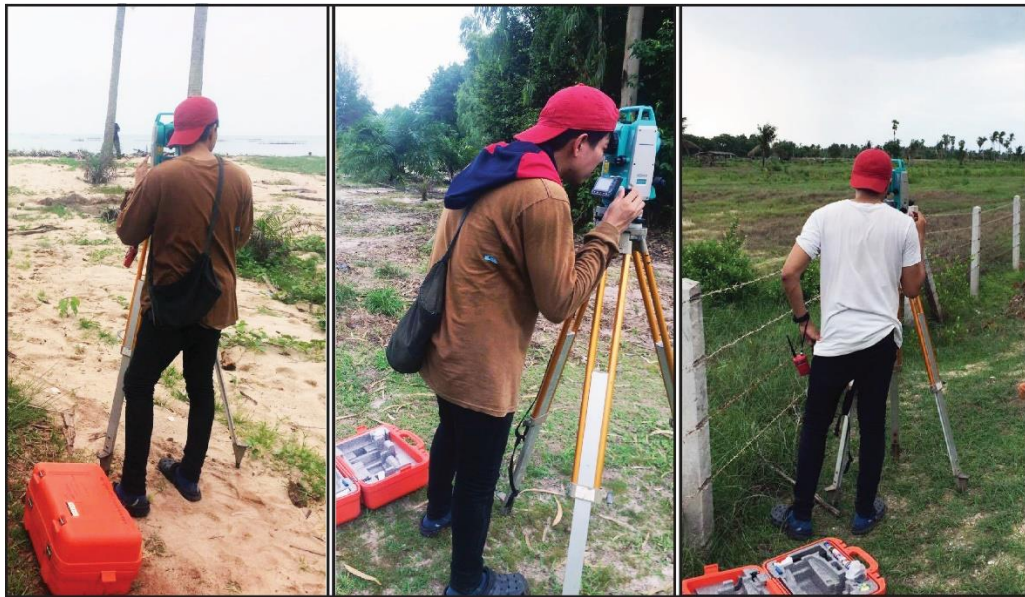
Figure 3.4 Total station survey camera measuring topographic profile along measurement at the study area.
