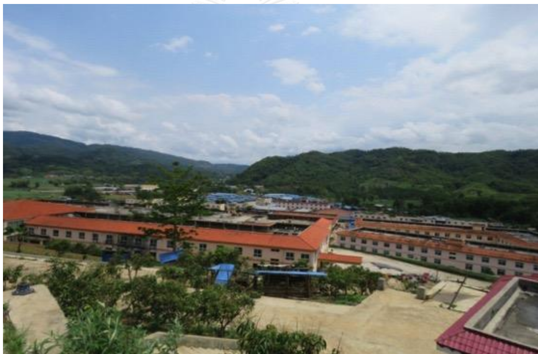
Figure 16. This is Lana Zup Ja Development Zone building (foreground) in which IDPs previously stayed for almost two years and in which some still stay. The majority of IDPs are now living in the new buildings with blue roofing (in the background). (Photograph by researcher, 19 May 2016).
