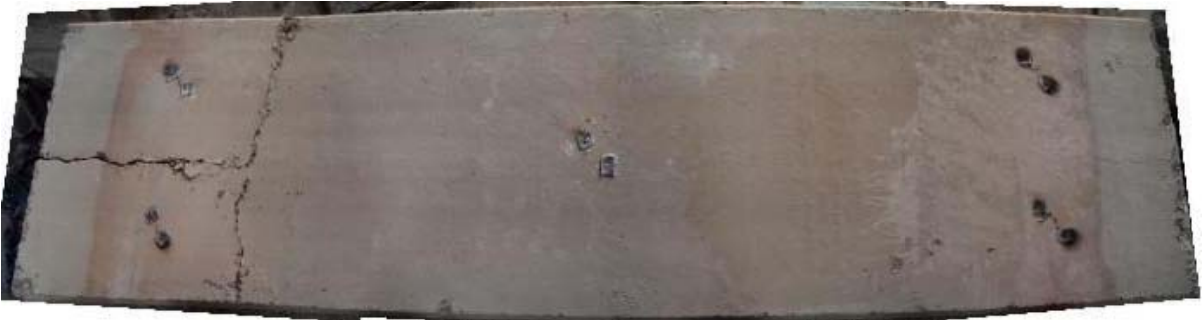
Figure 3.22 LB04 after fire test
