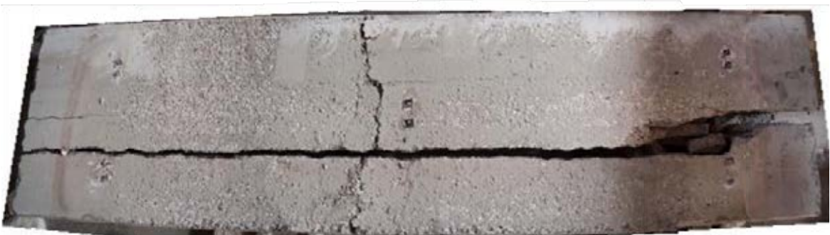
Figure 3.23 LB05 after fire test
