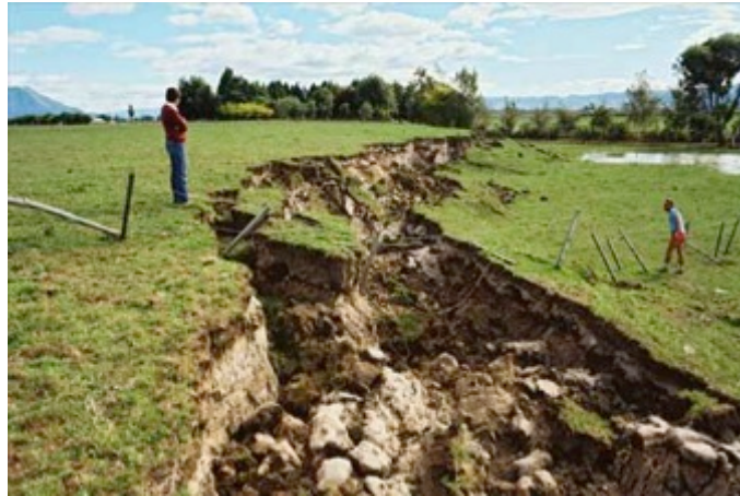
Figure 1.3 The effect of 1987 Edgecumbe earthquake. The land to the northwest of the Edgecumbe Fault sank by up to 2 meters. The fault ruptured the surface, forming a seven-kilometer-long rift across the countryside, and causing widespread damage from shaking.
