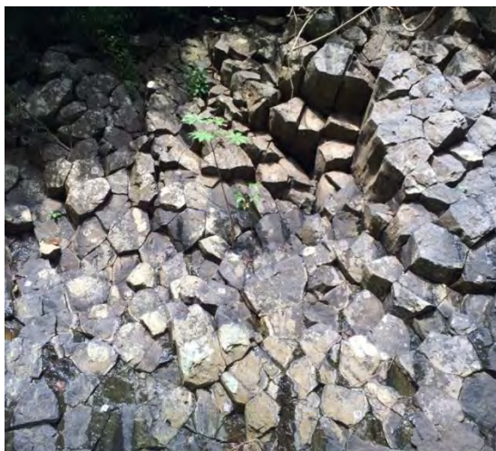
Figure. 24 Column tilted at same angle
