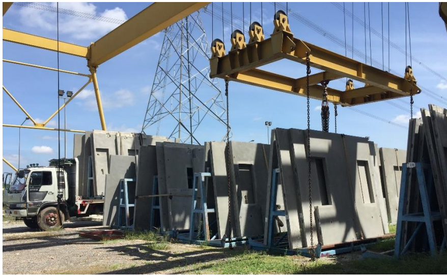
Figure 5 A-Frame racks in outdoor stockyard
