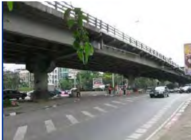
Figure 1.1 Composite I-girder bridges at intersections in Thailand
