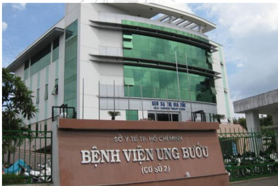
Figure 2: Oncology Hospital in Ho Chi Minh City(45)
