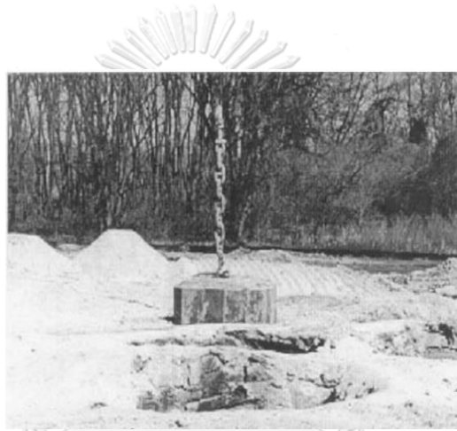
Figure 2.10. Dynamics compaction method (Kumar, 2001)
