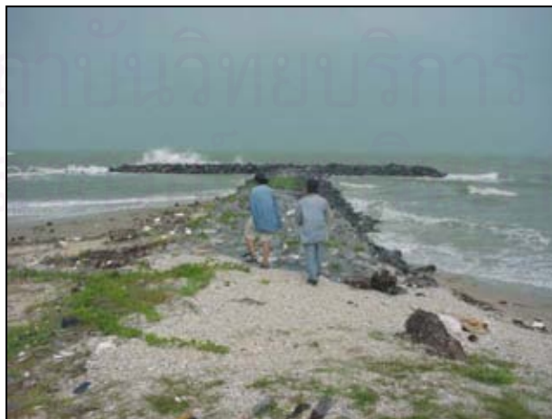
Figure 4.8 Groin T pattern at Ban Kho Phi, Kha Nap Nak sub-district, UTM 642216E/906809N
