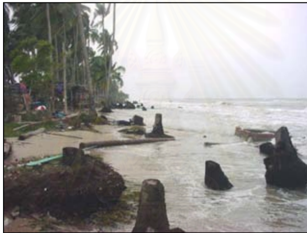
Figure 4.16 Eroded area at Ban Kong Kong, East, Pak Phanang sub-district UTM 636223E/ 927222 N shows coconut farm had destroyed
