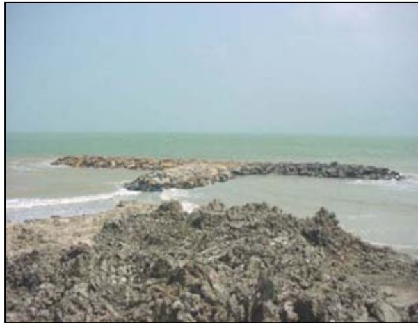
Figure 4.6 Groin T pattern at Ban Na Sarn, Na Saton sub-district, UTM 645698E/887542 N
