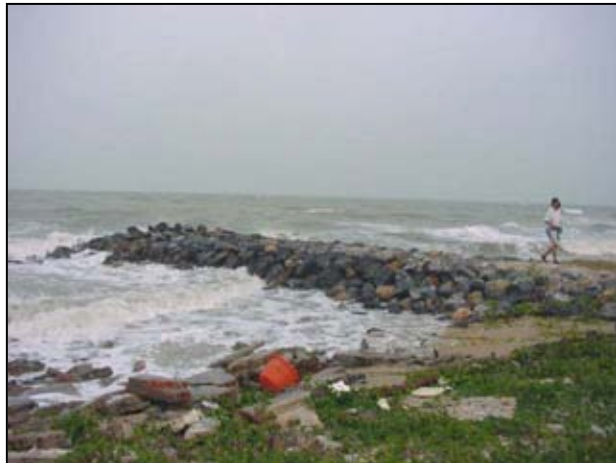
Figure 4.9 Groin I pattern at Ban Kho Phi, Kha Nap Nak sub-district, UTM 641910E/908326N
