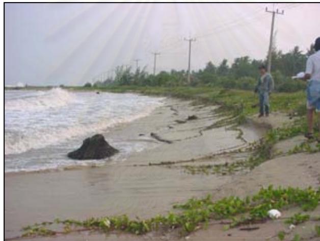
Figure 4.19 Eroded area at Ban Kho Fai, Kha Nab Nak sub-district UTM 641956E/907902N
