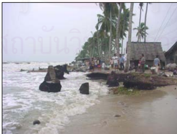
Figure 4.17 Eroded area at Ban Kong Kong, East, Pak Phanang sub-district UTM 636223E/927222N shows road, house and coconut tree had destroyed
