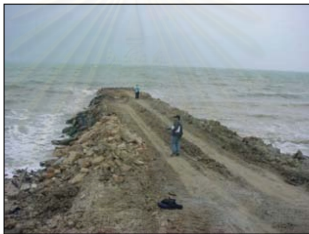
Figure 4.7 Groin I pattern at Ban Na Sarn, Na Saton sub-district, UTM 645635E/887795N
