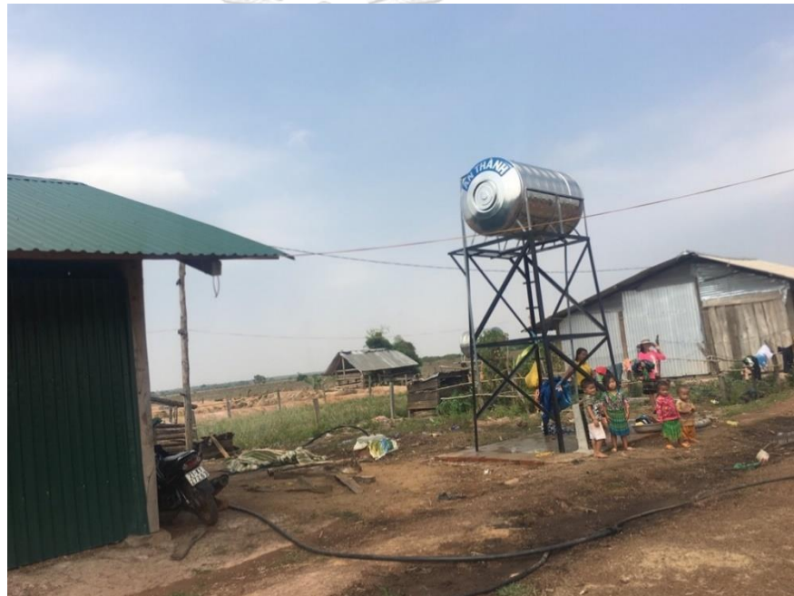
Figure 19: The water tank got install for the resettlement areas
