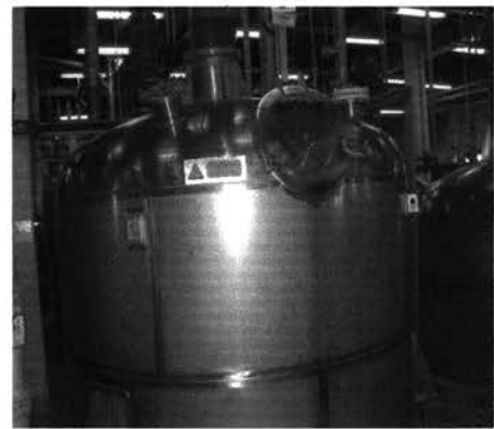
Neutral base in storage tank
