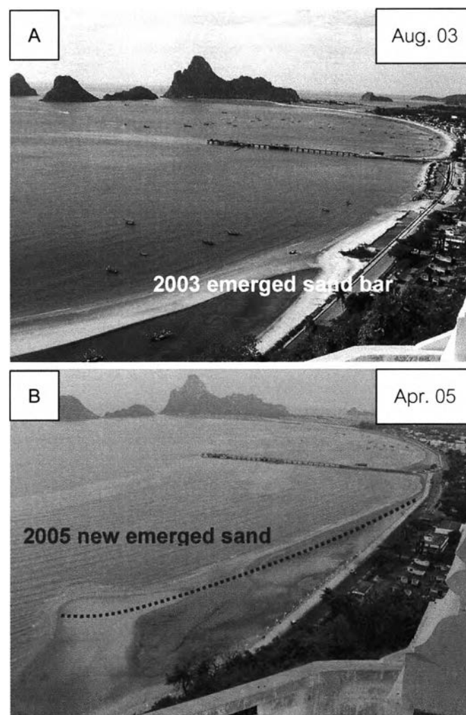
Figure 4.26 The photographs showing sediment movement in the area during low tide period. Both pictures were taken to the south of Prachuap Khiri Khan Bay. From picture A (taken on Aug 03), the sediments were moved by longshore current to the north (brown arrow), provided new sand bar.
