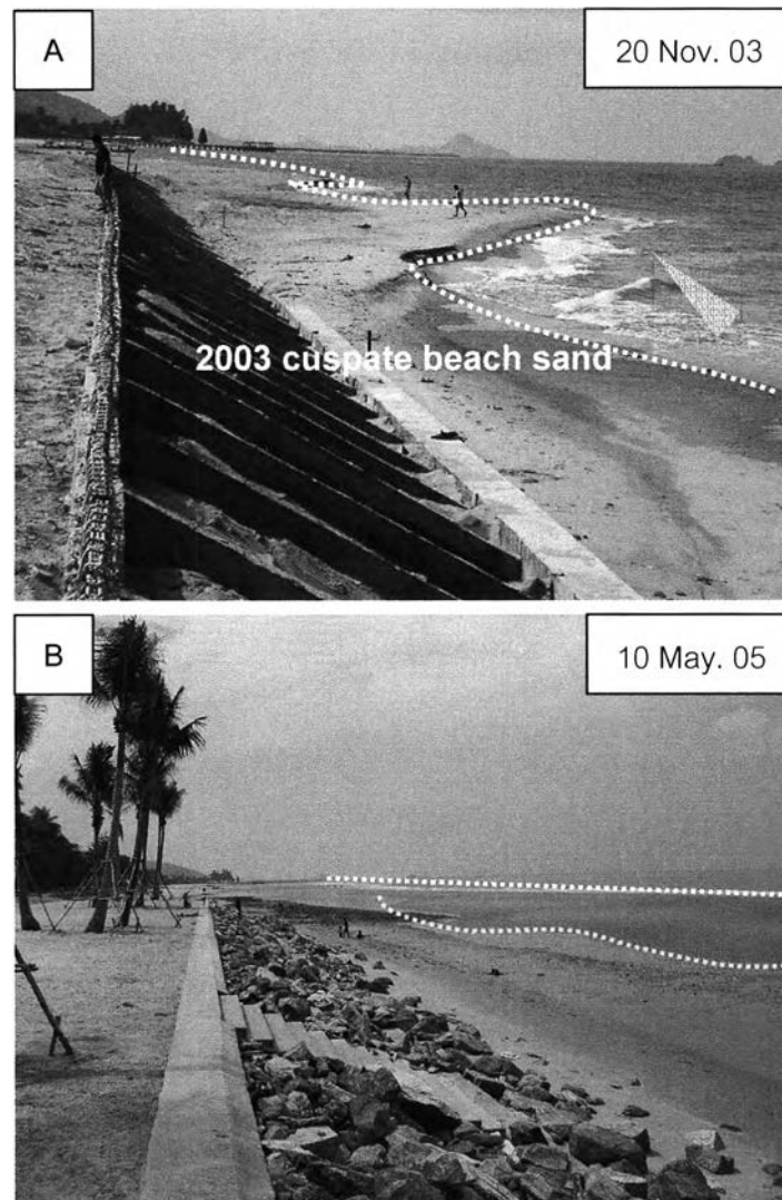
Figure 4.13 Photos showing the pattern of sediment accretion in the Pranburi area (UTM grid reference 609250N, 1367850N). Picture A is the pattern of cusped beach sand (white dot in picture A taken on 20 Nov 03 in low tide period). Sediments accrete along the beach barrier by the north longshore current. Picture B shows the developing of emerged sand bar, and developed into back barrier lagoon (picture was taken on 10 May 05). Pattern of sediment transportation and beach geomorphology, indicated that the deposition is more than erosion in this area. The erosion may be occurred in high monsoon season only.
