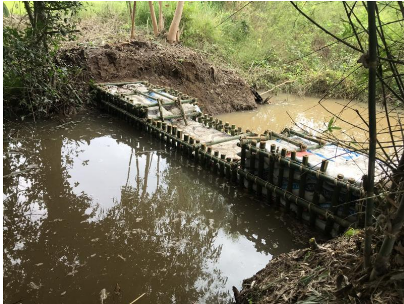
Figure 5.20 Weirs or water gates
