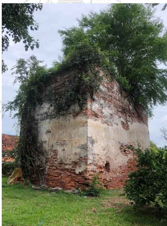
Figure 6.24 The remaining water tank.
