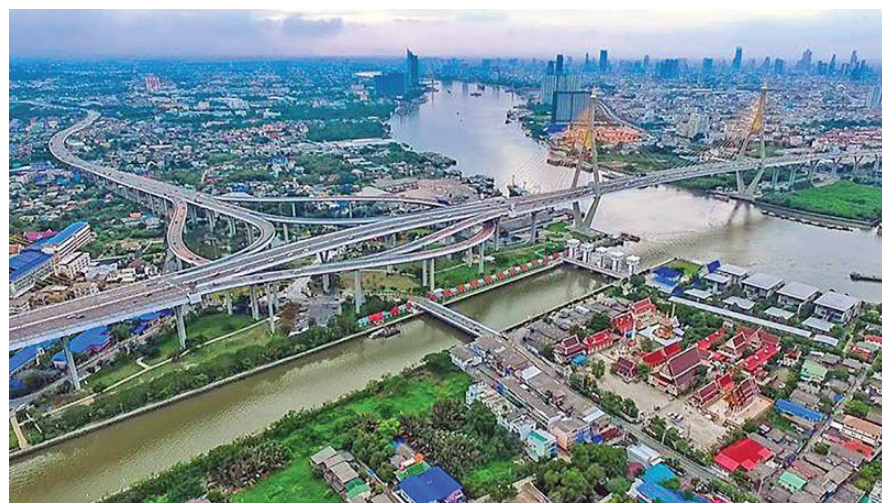
Figure 6.17 Khlong Lat Pho Irrigation Project.
