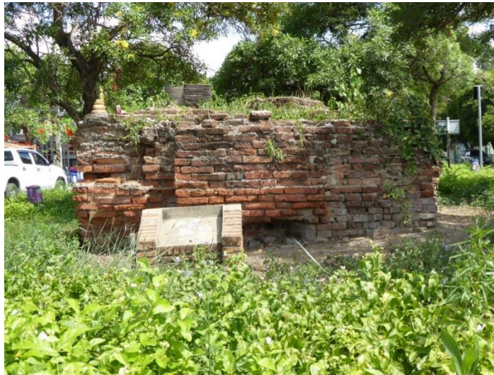
Figure 6.21 Shi kun Bridge.
