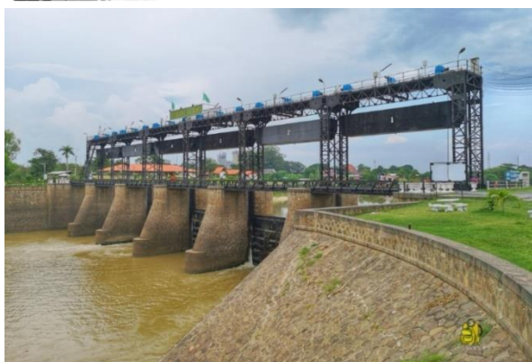
Figure 6.18 Rama VI Dam and its canal network.
