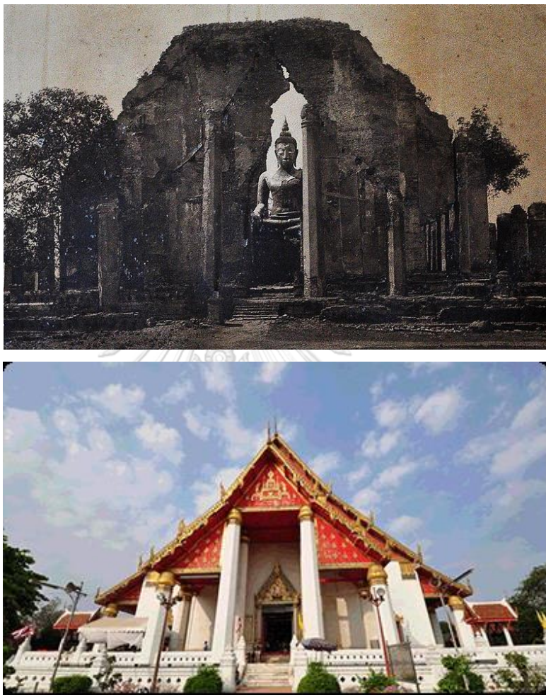
Figure 6.29 Mongkhonbophit Vihara before and after reconstruction
