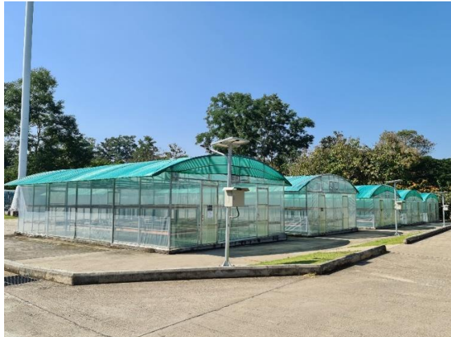
Figure 5: Image of Drying House
