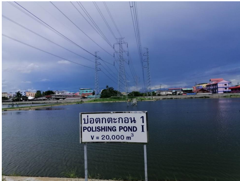
Figure D5 Sedimentation pond
