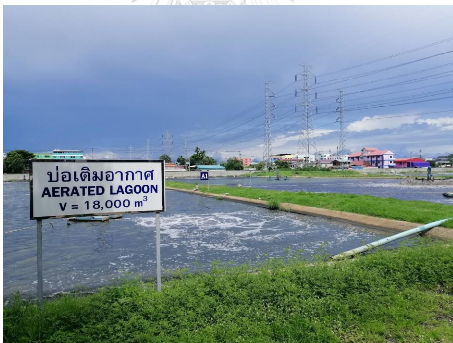
Figure D4 Aeration lagoon
