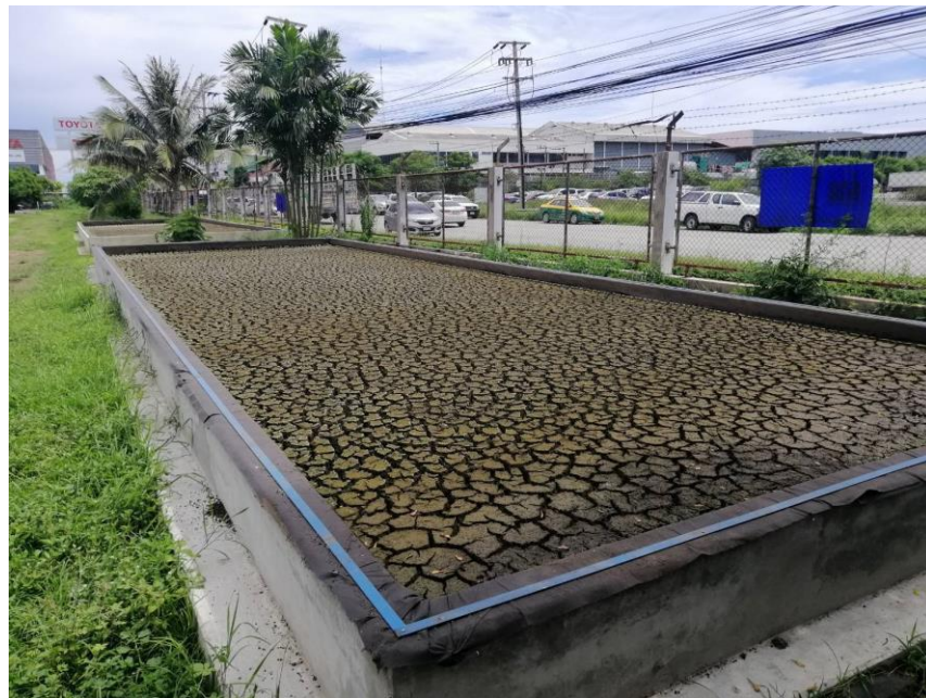
Figure D11 Sludge drying pond
