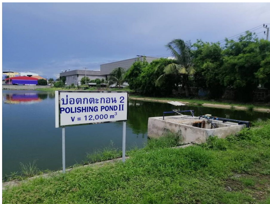
Figure D7 Sedimentation pond 2
