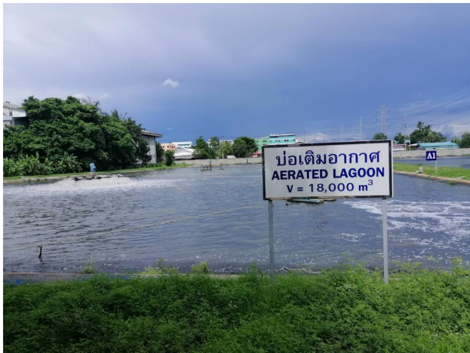
Figure D3 Aeration lagoon
