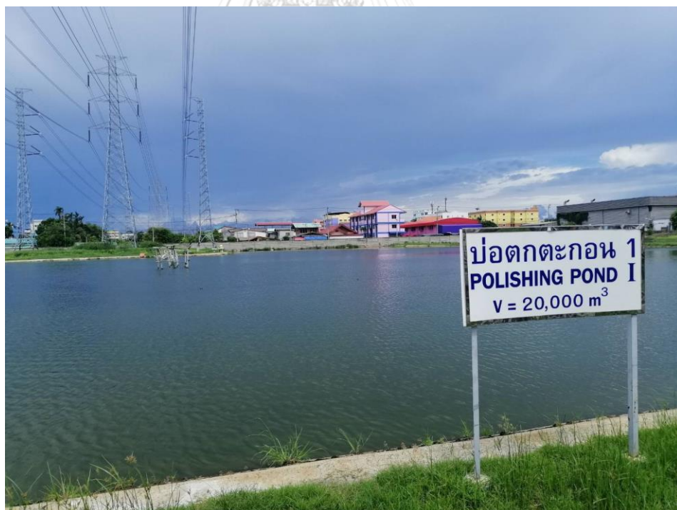
Figure D6 Sedimentation pond
