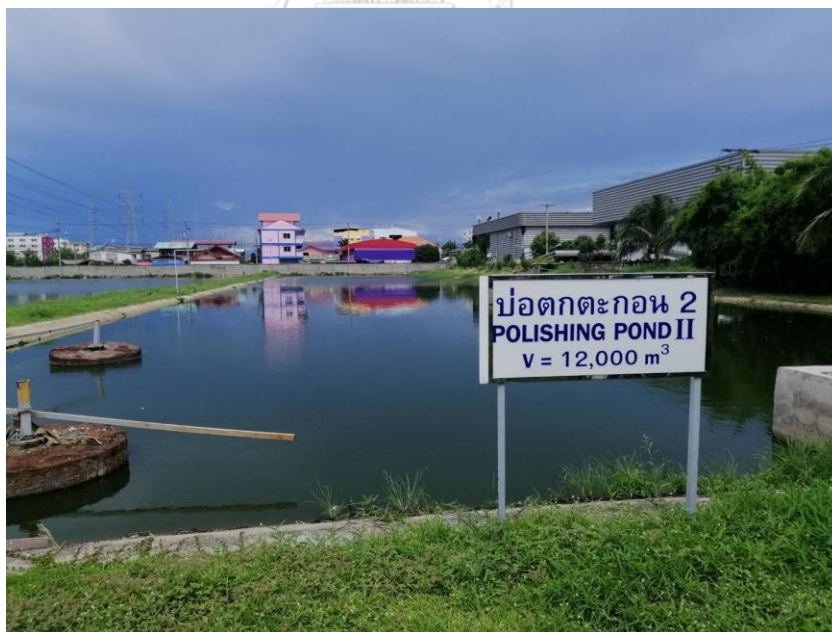
Figure D8 Sedimentation pond 2
