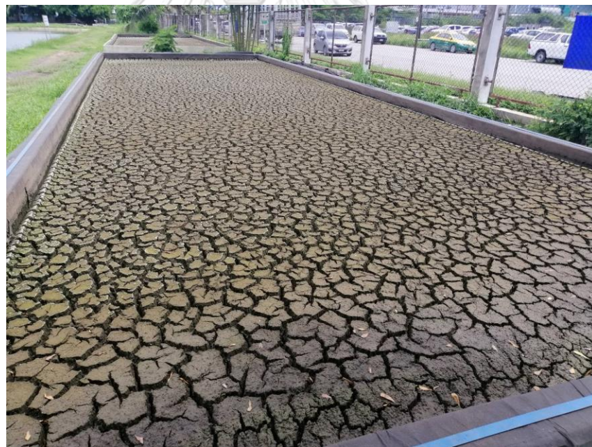
Figure D12 Sludge drying pond
