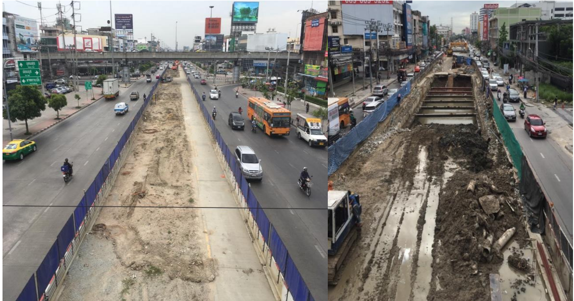
Figure 3.2 The on-road construction sites at (left) Srinagarindra road and (right) Pattanakarn
