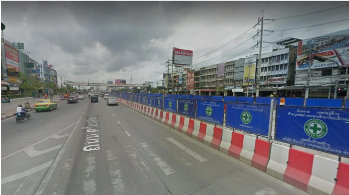
Figure 3.8 Srinagarindra sampling area at SRS
