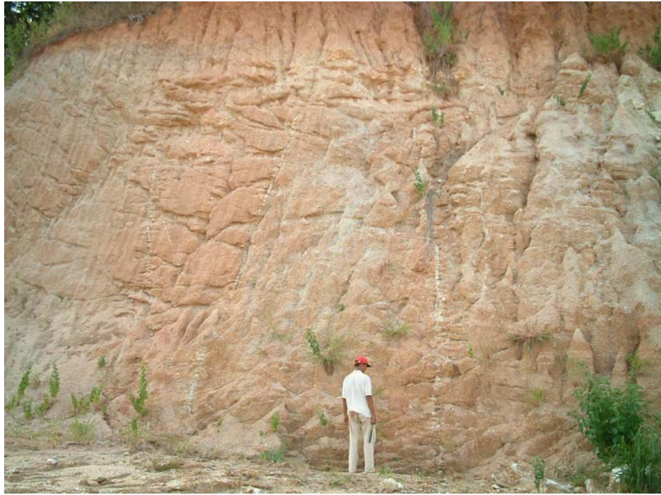
Figure 3.41 Exposure of highly weathered granite at Ban Klet Kaeo (Sattahip V). Grid reference 0707566 E 1408481 N.
