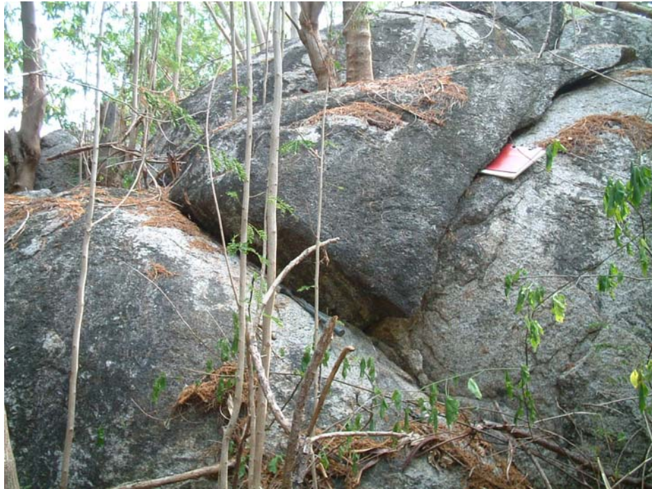
Figure 3.37 Exfoliated porphyritic granite at Khao Din in Bang Lamung area. Grid reference 0713747 E 1413877 N.
