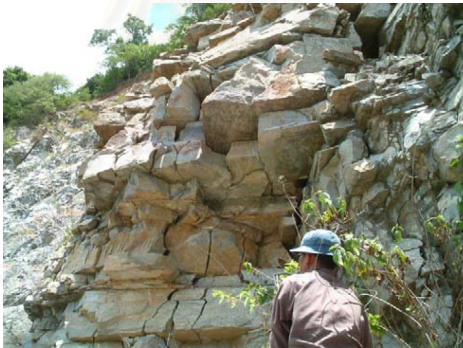
Figure 3.23 Gently NNE dipping bedded argillaceous limestone exposed at the southwestern part of Khao Plu Ta Luang. Brittle fractures are commonly observed. Grid reference 0713296 E 1403793 N.
