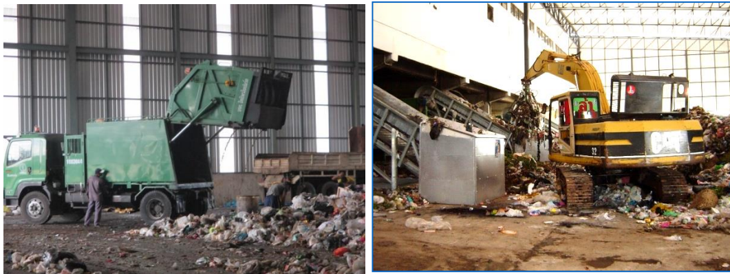
Figure 11 The Operation process at On-Nuch disposal plant
