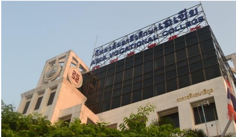
Figure 9.0: The building of the Asia Vocational College in Bangkok, Thailand.
