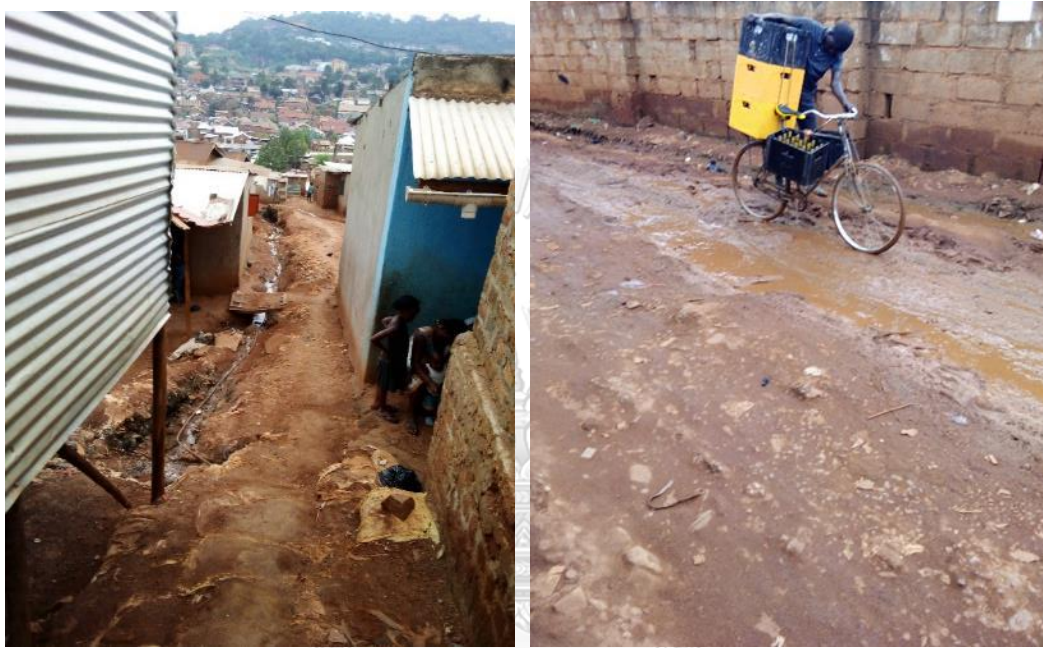
Figure 11: A typical road and a pathway in a moderately sized pathway in Kinawataka slum.
