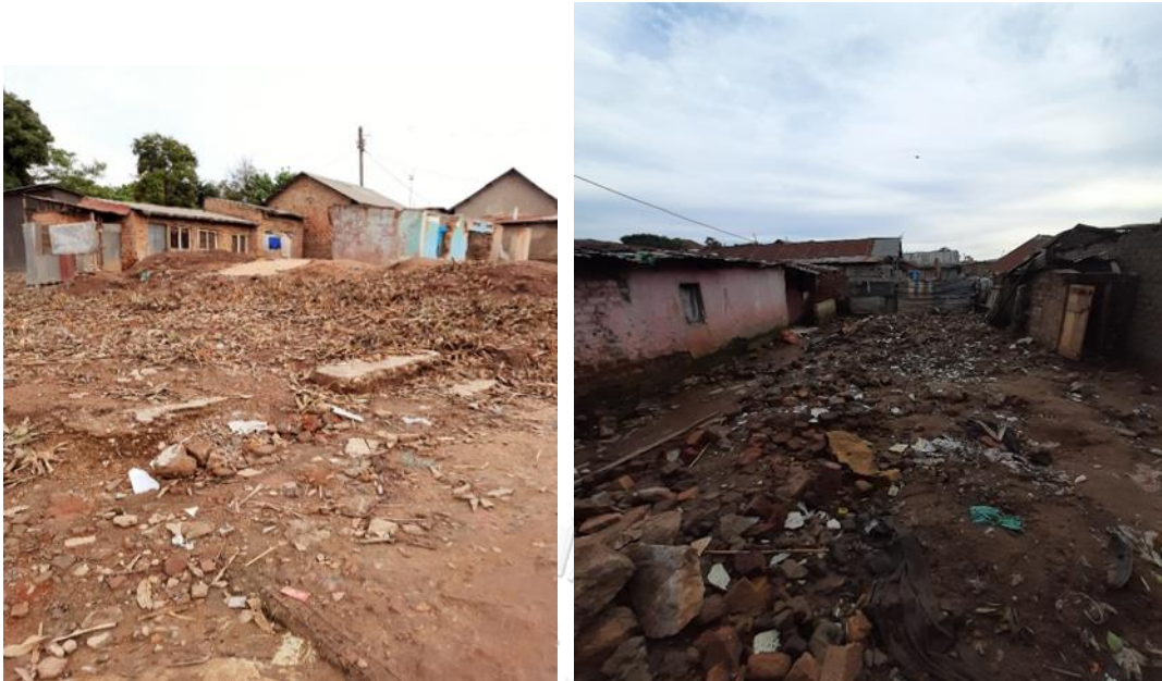
Figure 7: Picture showing evicted land in Ggaba Slum.
