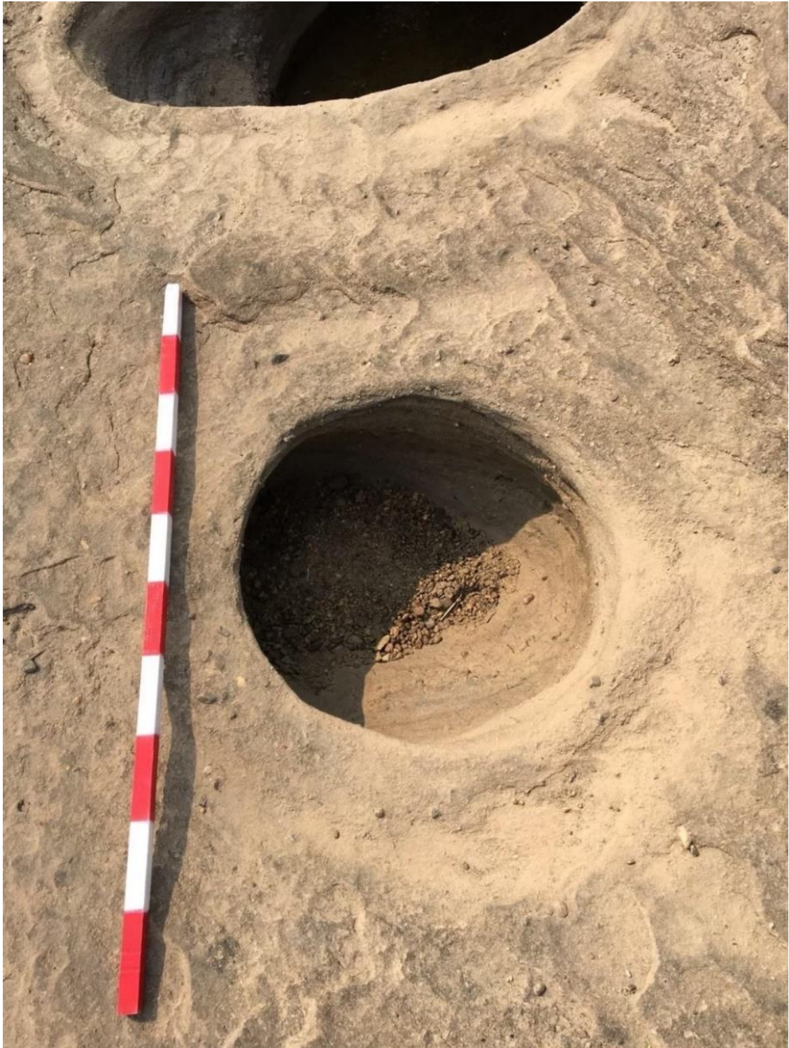
Figure 3.4 The image depicts the process of measuring the size and shape of a pothole.
