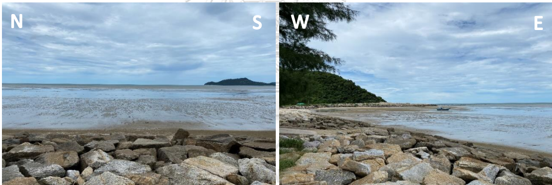
Figure 36. Pictures of the coast at Station 6, a riprap revetment was found at the coast.
