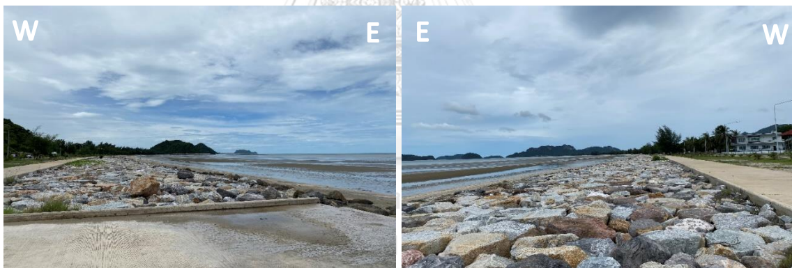
Figure 38. Pictures of the coast at Station 7, a riprap revetment and seawall were found at the coast.
