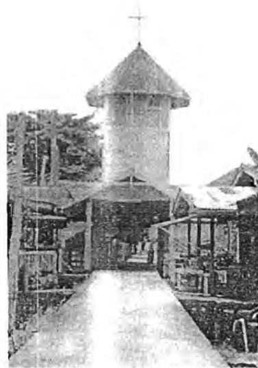
Figure 5. The bell tower
