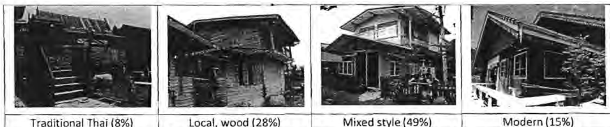
Fig. 1: Types of houses in the Soi Wat Lung Ban Community Source: Kaengtonglang, 2011
