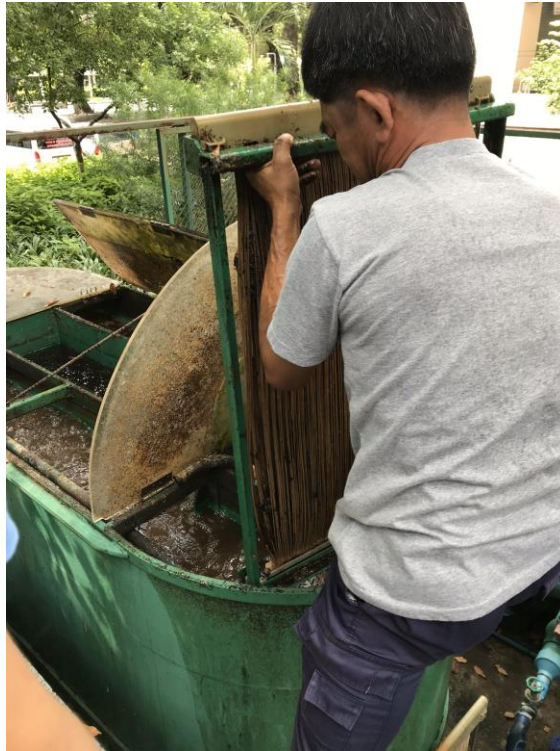
Figure 26 Moving the MBR for cleaning
