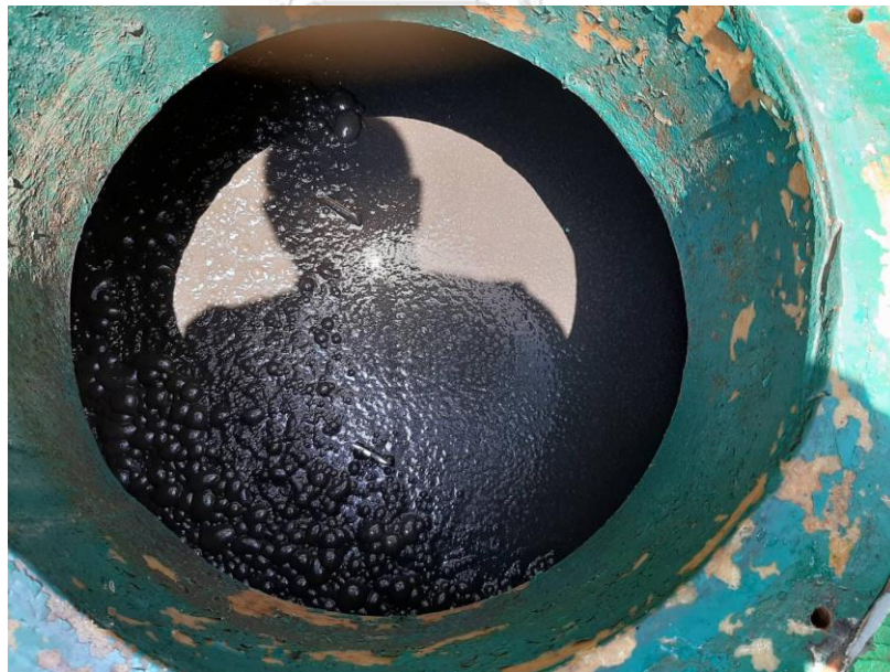
Figure 20 The anaerobic digester that is filled by the swine manure at the beginning stage of the zero-waste system
