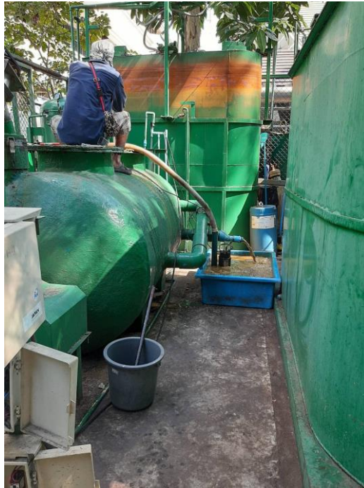
Figure 19 Swine manure is loaded into the digester
