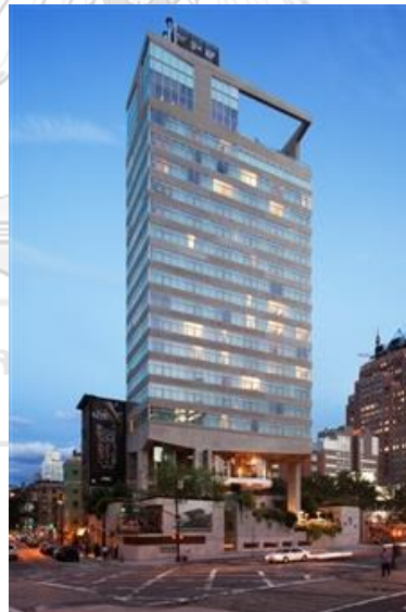
Figure 1.3 The James Building, New York
