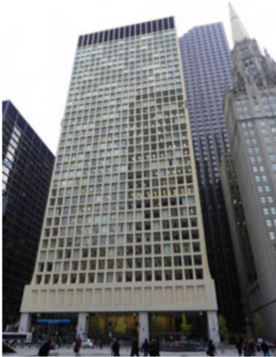
Figure 1.4 The Brunswick Building, Chicago, Illinois
